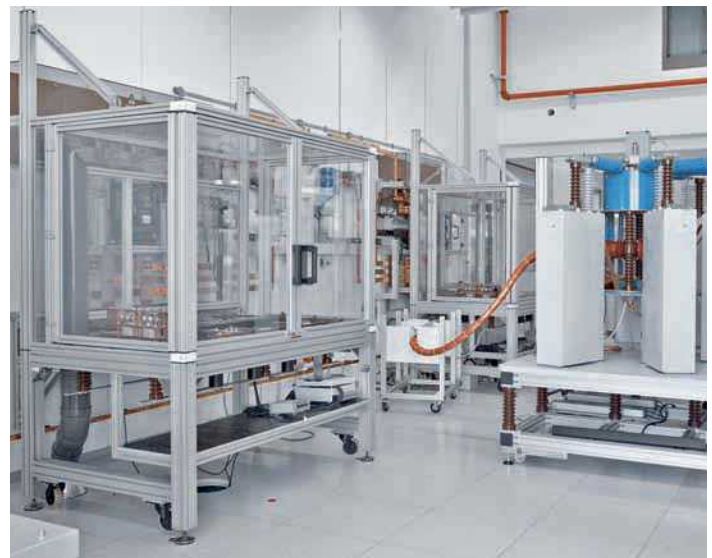
Fig. 24: Testing stations of the high-current testing system
