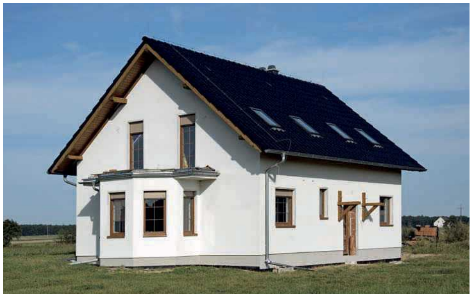
Fig. 15 External lightning protection, on the outside of a private residence, for example
