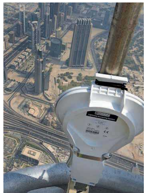
Fig. 34: Burj Khalifa, LM-S application
