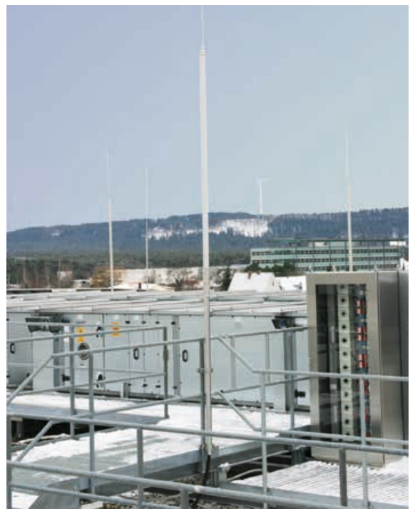
Figure 5.2.4.10 Installation of a HVI power Conductor
