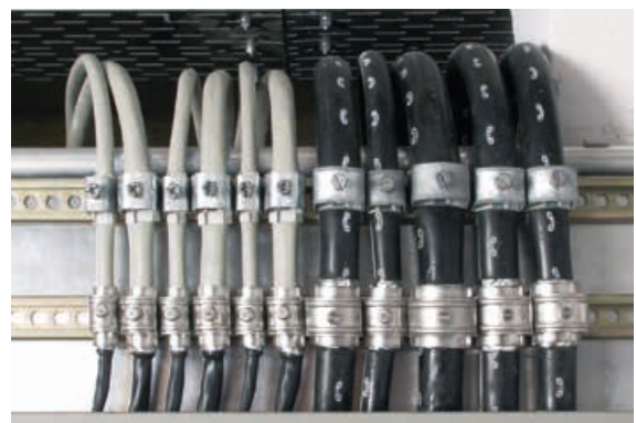
Figure 6.3.4 Lightning current carrying shield connection system (SAK)
