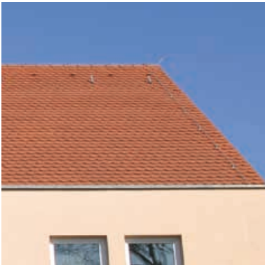
Figure 5.1.2.1 Air-termination system on a gable roof
