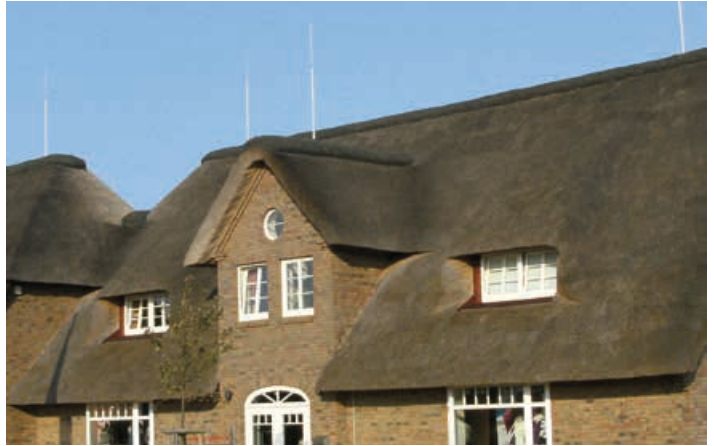
Figure 5.1.5.4 Historical farmhouse with external lightning protection system; source: Hans Thormählen GmbH & Co.KG.
