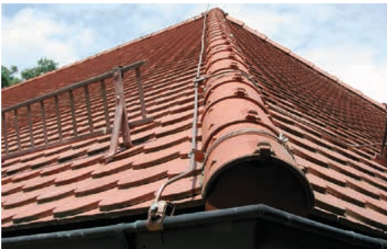
Figure 5.1.1.18 Gable roof with conductor holder
