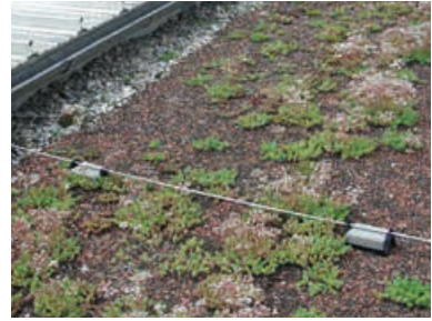
Figure 5.1.7.3 Conductor routing above the cover layer
