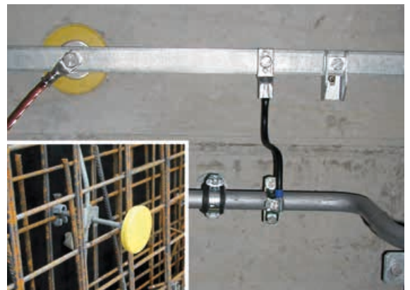
Figure 5.5.2.5 Fixed earthing terminal
