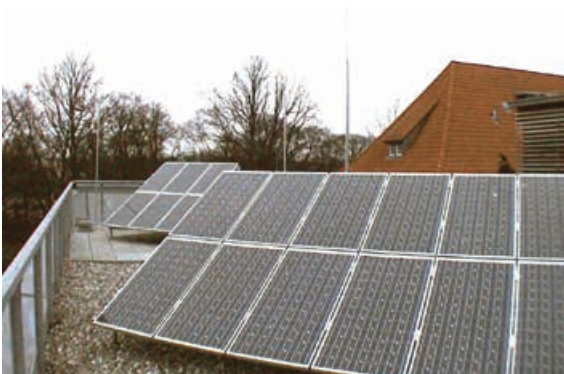
Figure 5.1.8.6 Isolated air-termination system of a photovoltaic system
