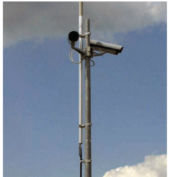
Figure 9.22.4 HVI Conductor installed at a pylon
