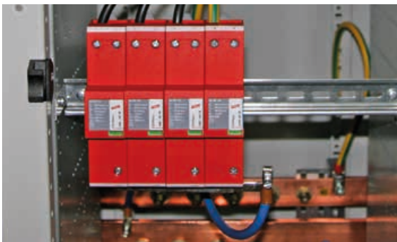
Figure 9.16.8 Coordinated type 1 surge arrester
