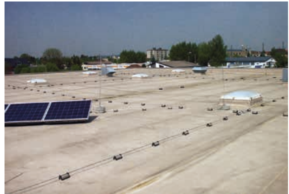
Figure 5.1.3.2 Practical use of air-termination rods
