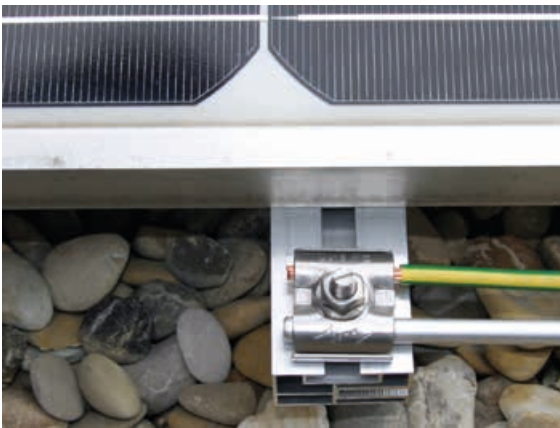
Figure 9.18.3 UNI earthing clamp: A stainless steel intermediate element prevents contact corrosion, thus establishing reliable long-term connections between different conductor materials
