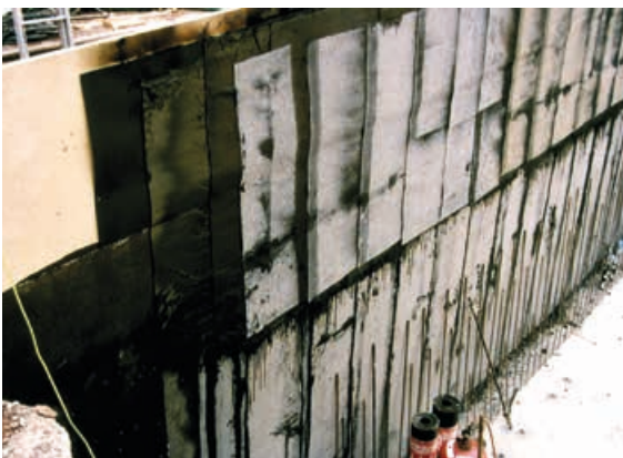
Figure 5.5.2.18 Bituminous sheetings used as sealing material
