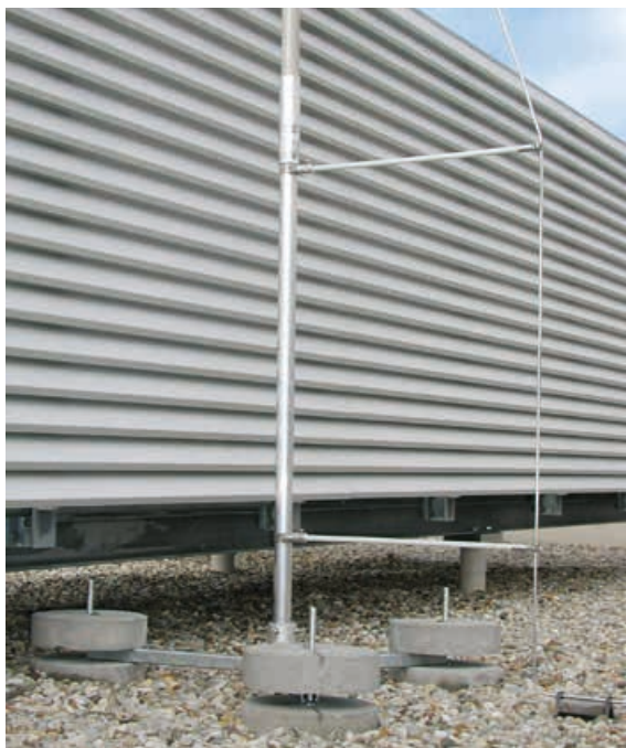
Figure 5.1.8.10 Tripod for isolated supporting tubes
