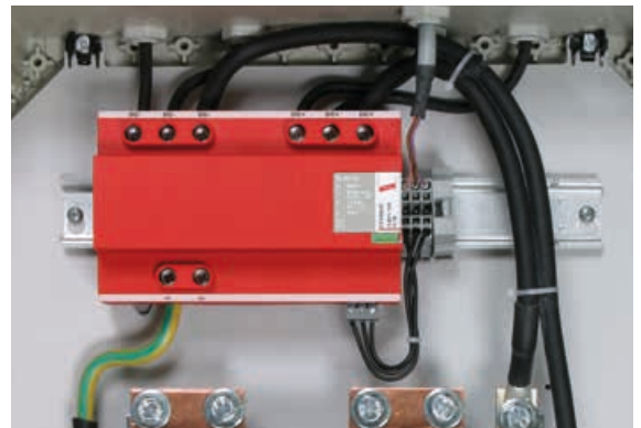
Figure 9.18.8 DEHNlimit PV 1000 V2 spark-gap-based type 1 combined arrester
