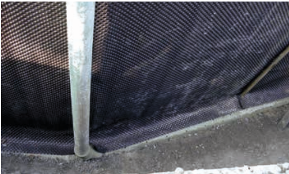
Figure 5.5.2.11 Use of dimpled membranes
