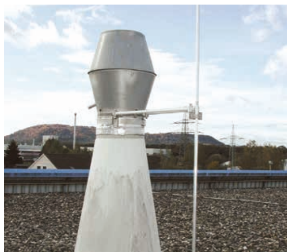
Figure 5.1.8.3 Air-termination rod with spacer
