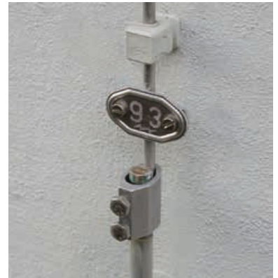
Figure 5.2.2.3.1 Test joint with number plate
