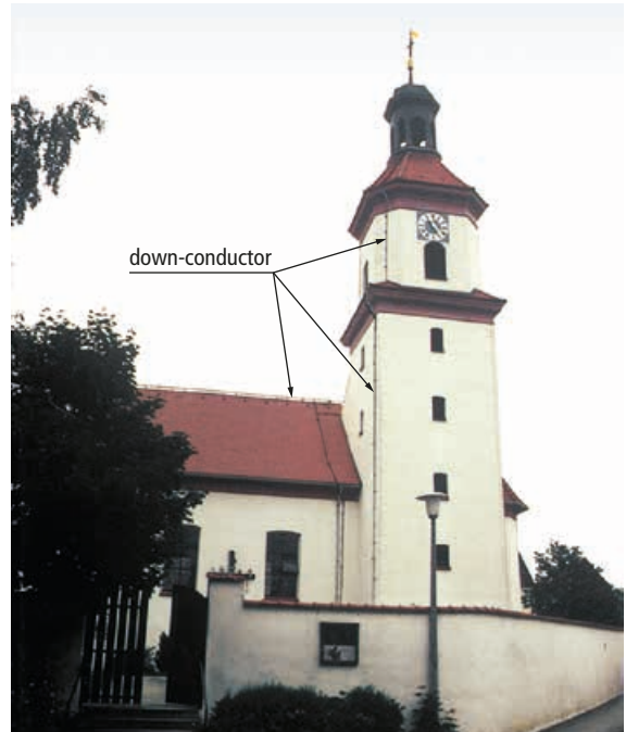
Figure 5.1.9.1 Installation of the down conductor on a steeple
