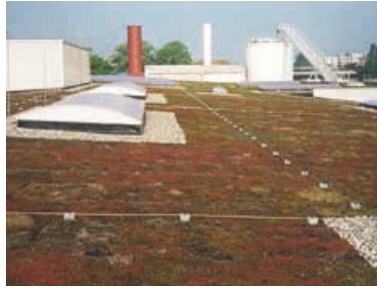
Figure 5.1.7.2 Air-termination system on a green roof
