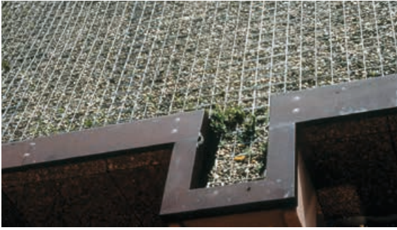
Figure 7.3.7a Galvanised reinforcement mats for shielding the building
