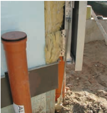
Figure 5.2.2.2.3 Earth connection of a metal façade
