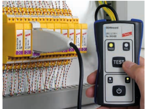
Figure 8.2.6.2 LifeCheck arrester testing by means of DRC LC M1+
