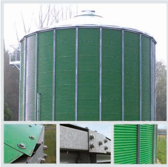
Figure 9.3.6 Fermenter made of bolted metal sheets
