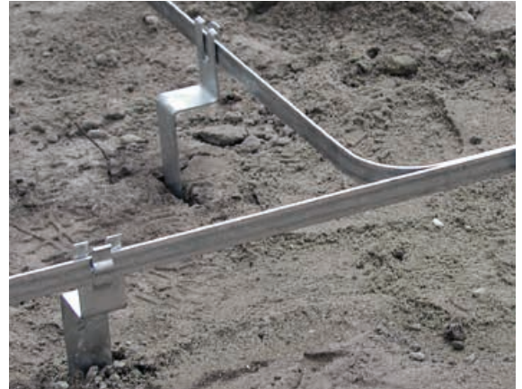
Figure 5.5.2.3 Foundation earth electrode
