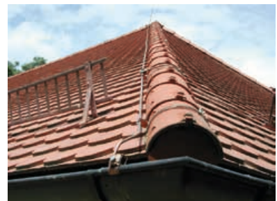
Figure 5.2.2.1.3 Air-termination system connected to the gutter
