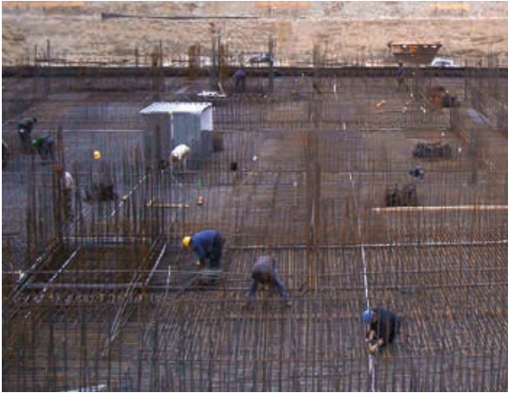
Figure 5.5.2.6 Meshed foundation earth electrode
