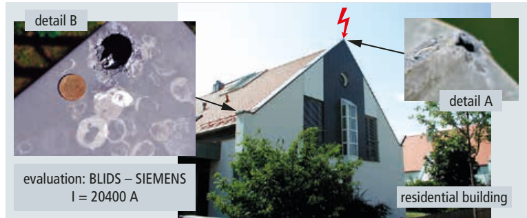
Figure 5.1.4.2 Example of damage: Sheet metal
