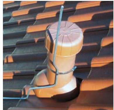
Figure 5.1.2.3 Additional air-termination system for vent pipes
